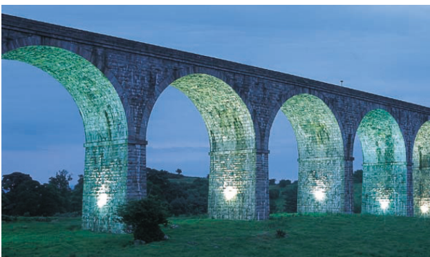
Viaduct and Rail Line, Newry and Mourne District Council. Source: Newry and Mourne District Council
